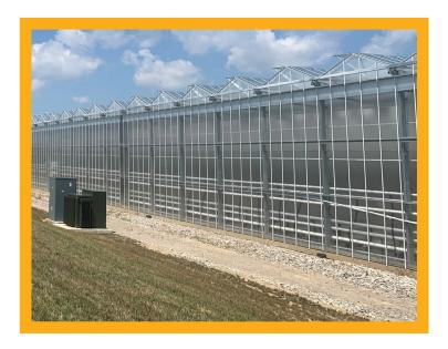
achieve optimal light intensities. Because of the height and glass roof, the Venlo style structure requires less maintenance than other standard greenhouse structures, leading to decreased operating expenses.
