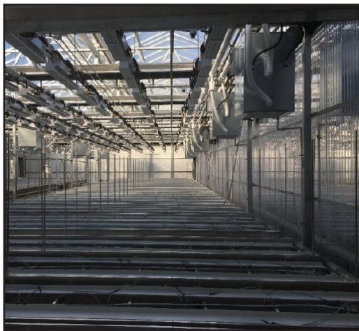
Example and schematic of overhead fan coil units
